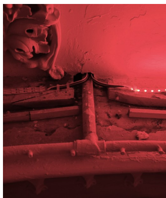
Gas nozzle extending from the ring of gas jets to the attic side of the dome.
